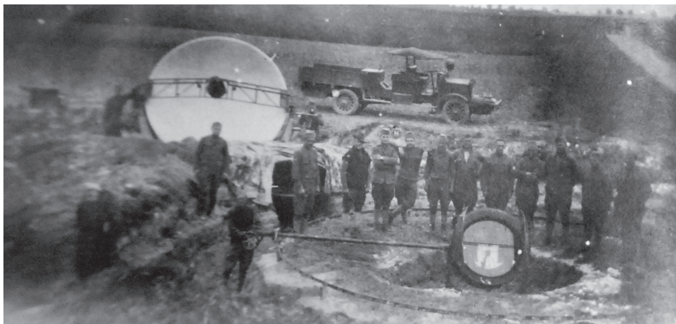
American searchlight crew and equipment in action on Somme front. 36" searchlight of high power showing arrangement of digging in for protection, also camouflaged earth works, plotting room and paraboloid sounding device for locating approaching planes by sound. Large Riker truck with generator built in front. Position near Gleeszy. Morris' War Photographs. Courtesy of the Library of Congress.
