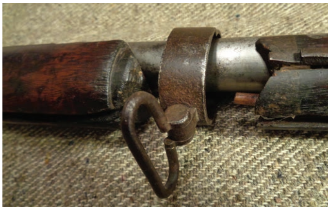
FIG 13. In order to disguise the Needham conversion rifles, the stocks were cut on many of them, so they could be shipped to the Vermont/Quebec border in small crates. Courtesy of the author.
